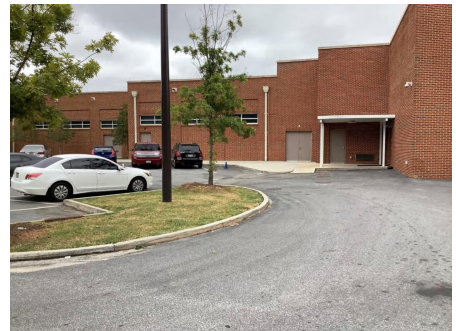
9). North Elevation - Dec 04, 2019
