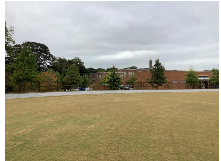
6). Northwest Elevation - Dec 04, 2019
