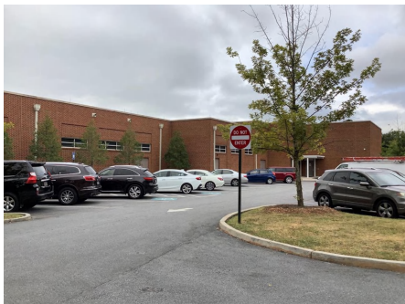
10). North Elevation - Dec 04, 2019
