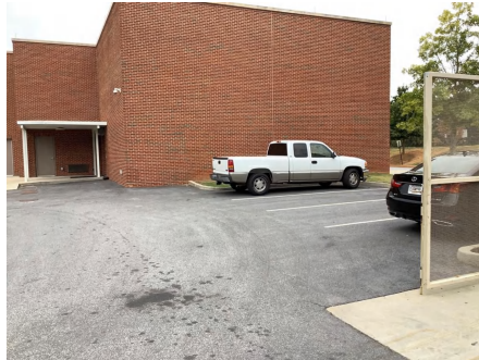
8). Northwest Elevation - Dec 04, 2019
