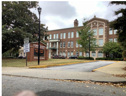
8). Northeast Elevation - Dec 04, 2019
