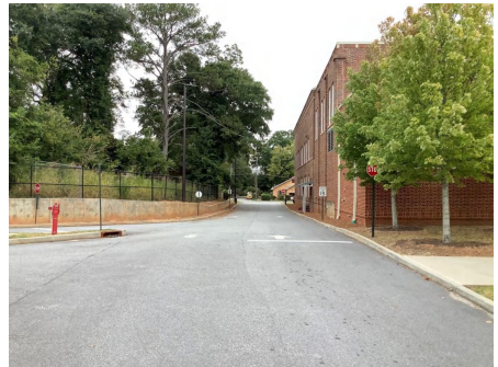
6). Northwest Elevation - Dec 04, 2019
