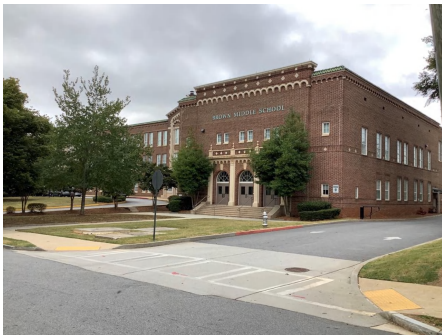
7). Northeast Elevation - Dec 04, 2019
