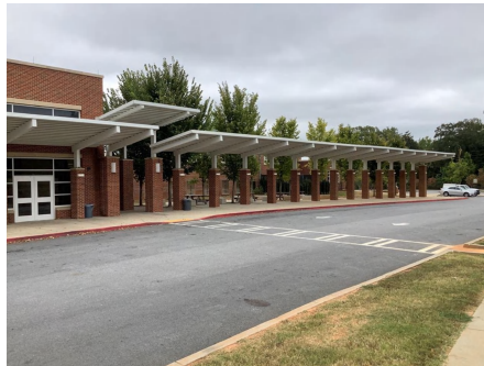
5). West Elevation - Dec 04, 2019
