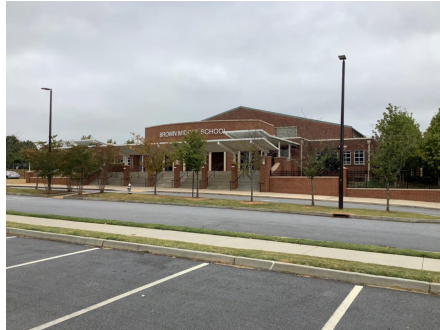
2). South Elevation - Dec 04, 2019
