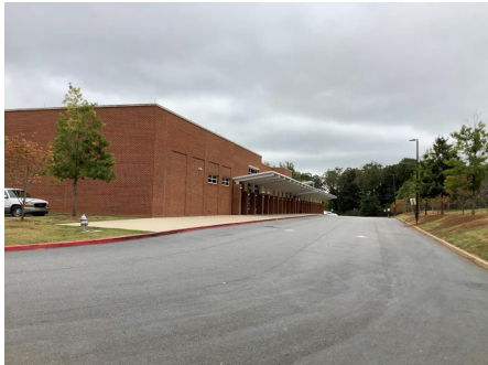
7). Northwest Elevation - Dec 04, 2019
