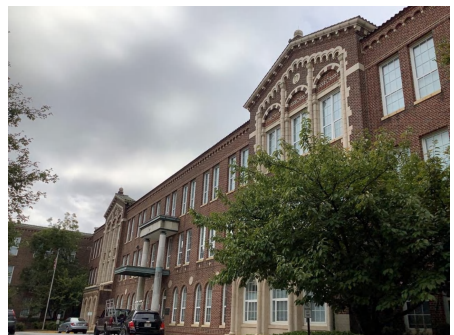
9). East Elevation - Dec 04, 2019
